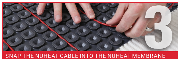
SNAP THE NUHEAT CABLE INTO THE NUHEAT MEMBRANE
