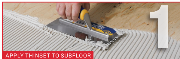
APPLY THINSET TO SUBFLOOR
