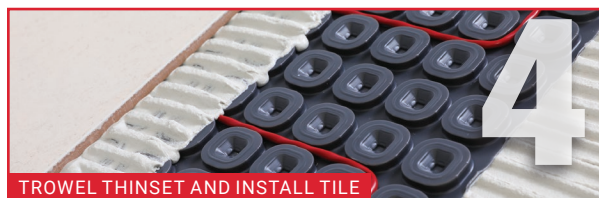
TROWEL THINSET AND INSTALL TILE
