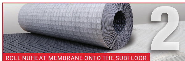
ROLL NUHEAT MEMBRANE ONTO THE SUBFLOOR
