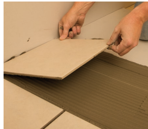
Trowel Thinset and Install Tile
