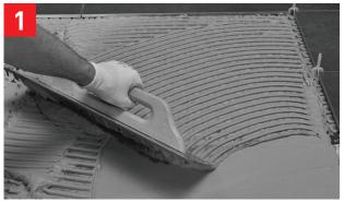
Apply an additional layer of thinset mortar on top using a notched trowel suitable for the tile type/size.
