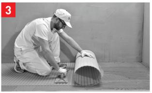
Press the **Nuheat Membrane** with a roller or a flat trowel.
