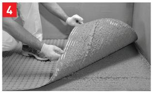
Check underside of **Nuheat Membrane** to ensure 100% thinset coverage.
