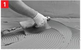
Spread a suitable thinset mortar to the substrate using a suitable trowel.
