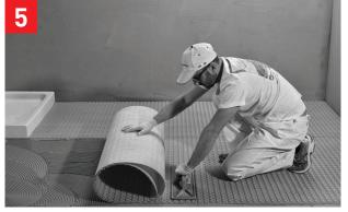
Lay down the next sheet of **Nuheat Membrane** and align it with the previous one without overlapping. Line up the pillars of **Nuheat Membrane** to facilitate the installation of the heating cable.
