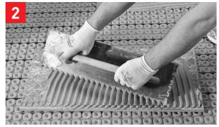
Apply thinset to the back of the tile using a notched trowel. Ensure 100% coverage especially with large format tiles. Lay the tile onto **Nuheat Membrane** and onto the fresh layer of thinset.
