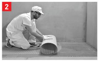
Roll Nuheat Membrane onto the thinset mortar.
