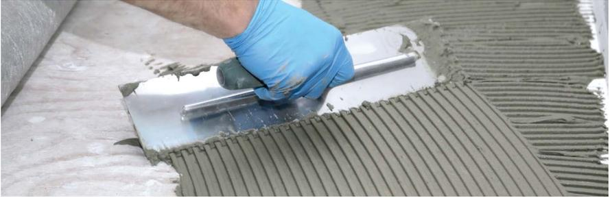
FIGURE 2.12: Spread thinset onto subfloor
