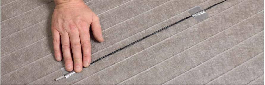
FIGURE 2.16: Secure floor sensor probe
