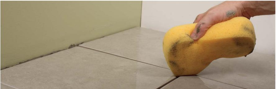
FIGURE 2.23: Clean grout lines
