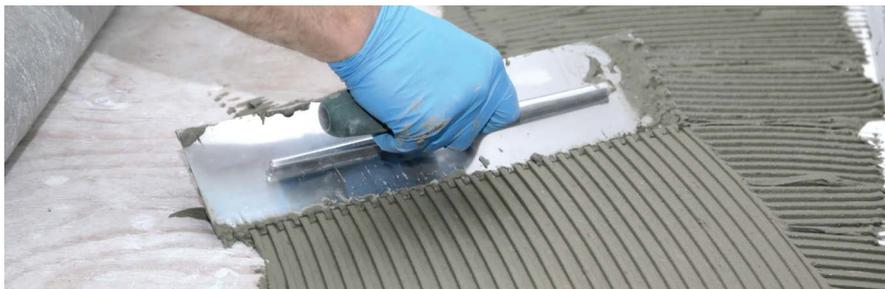
FIGURE 2.12: Spread thinset onto subfloor
