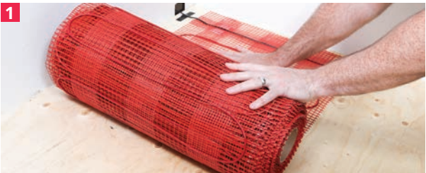
Roll out adhesive mesh
