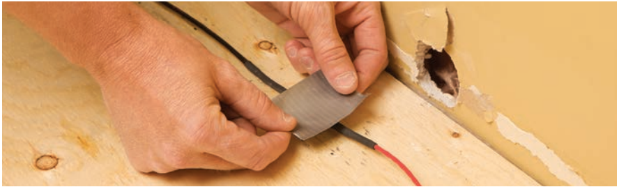
Figure 2.2.3: Secure the cold lead to the subfloor
