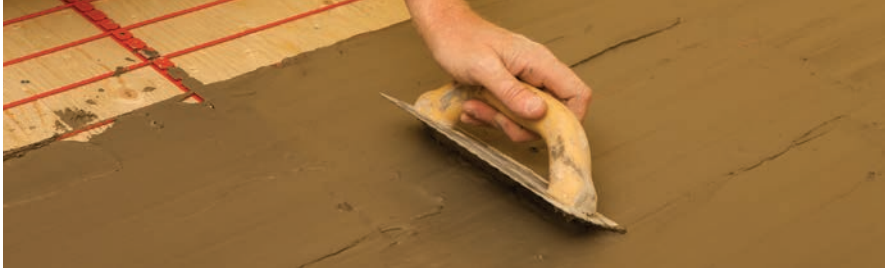
Figure 2.5.2: Thinset mortar method
