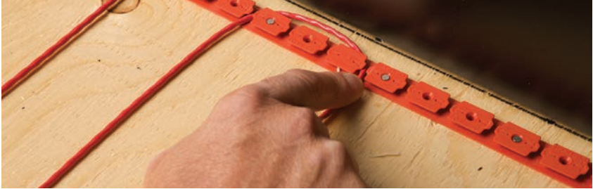
FIGURE 2.26: Install the heating cable
