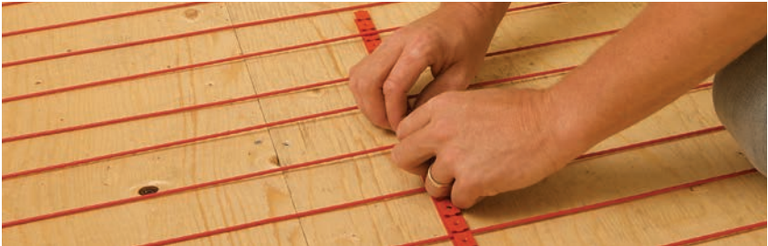
FIGURE 2.29: Install stabilizing guides
