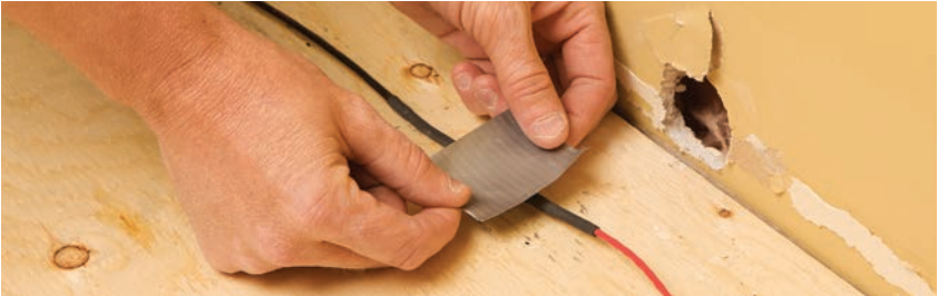
FIGURE 2.23: Secure the cold lead to the subfloor
