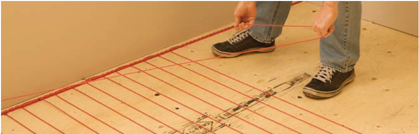
FIGURE 2.27: Install the heating cable
