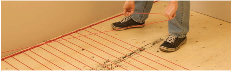
Figure 2.2.7: Install the heating cable
