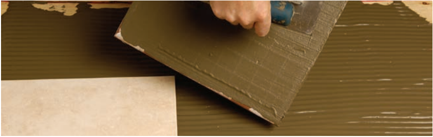
FIGURE 2.62: Direct method
