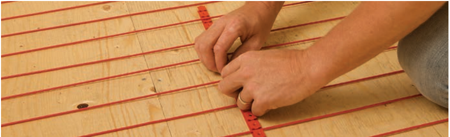
Figure 2.2.9: Install stabilizing guides
