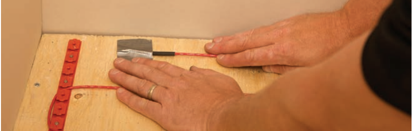
FIGURE 2.28: Secure the end seal
