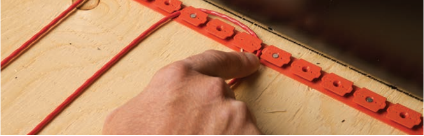
FIGURE 2.26 : Installer le câble chauffant
