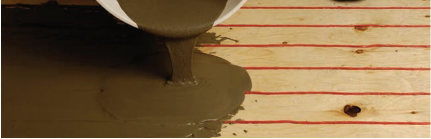
FIGURE 2.42: Self-leveling compound method
