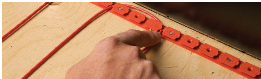
Figure 2.2.6 : Installer le câble chauffant
