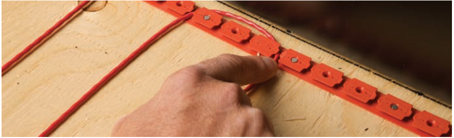
Figure 2.2.6: Install the heating cable
