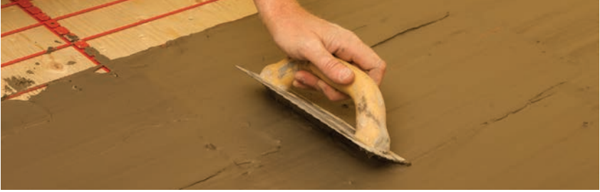
FIGURE 2.52: Thinset mortar method
