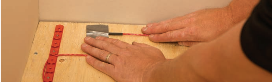
Figure 2.2.8: Secure the end seal
