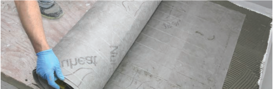
Place mat onto fresh thinset
