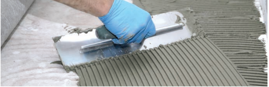
Spread thinset onto subfloor
