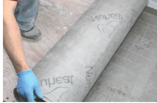
ROLL MAT ONTO THINSET
