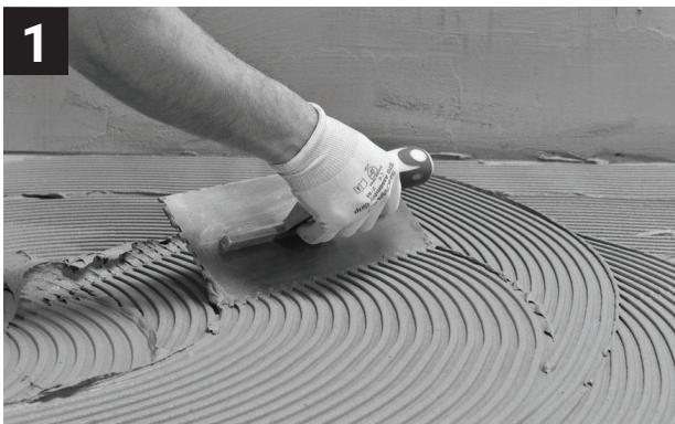
Spread a suitable thinset mortar to the substrate using a suitable trowel.
