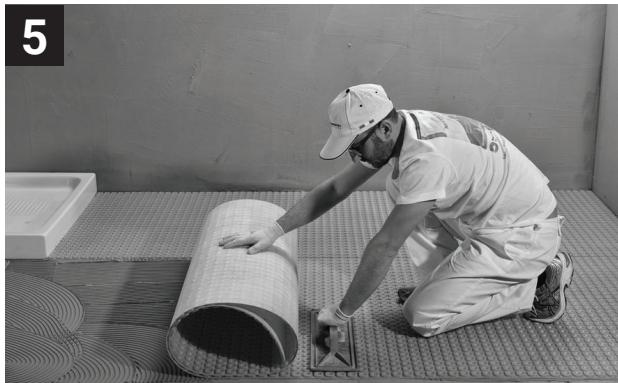
Lay down the next sheet of Membrane and align it with the previous one without overlapping. Line up the pillars of Membrane to facilitate the installation of the heating cable.
