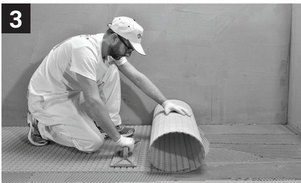
Press the Membrane with a roller or a flat trowel.
