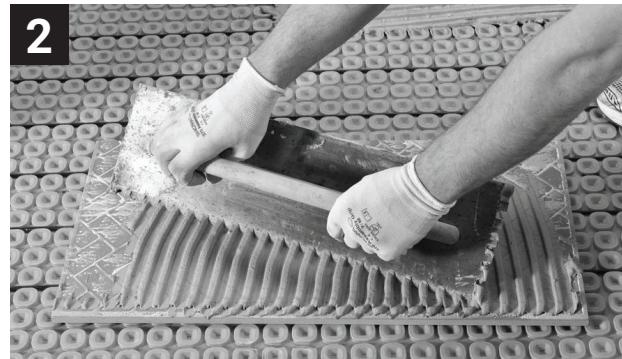
Apply thinset to the back of the tile using a notched trowel. Ensure 100% coverage especially with large format tiles. Lay the tile onto Membrane and onto the fresh layer of thinset.
