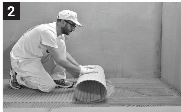
Roll Membrane onto the thinset mortar.
