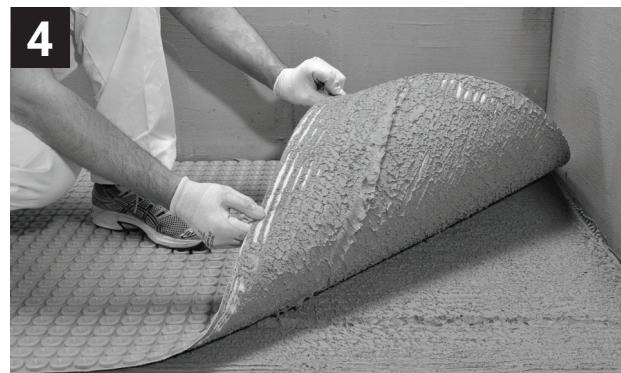
Check underside of Membrane to ensure 100% thinset coverage.
