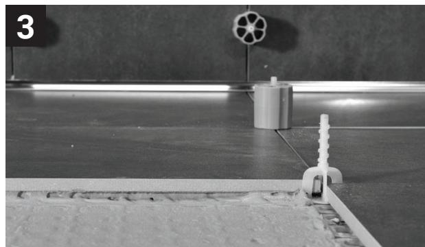
Carefully lay the tiles and press them on the layer of thinset. If a layer of skin has formed on the thinset, remove and apply again.
