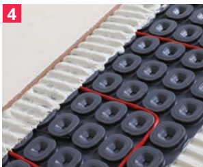
4 Install floor covering covering heated area
