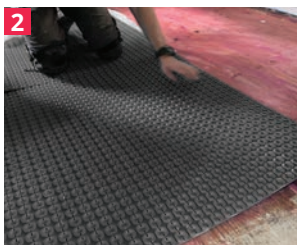
2 Press Peel & Stick Membrane onto substrate
