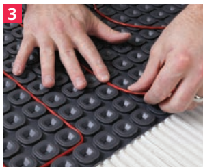
3 Route cable throughout heated area
