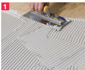
1 Apply thinset onto substrate
